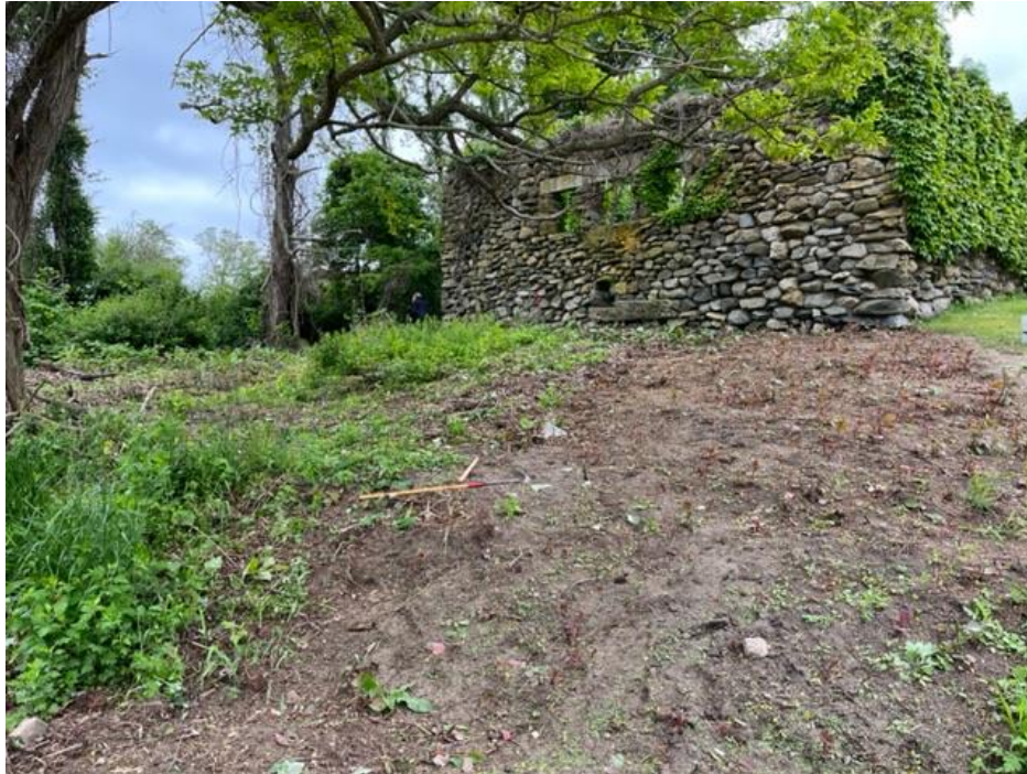
View of Sprague Stable ruin post-knotweed-clearing
